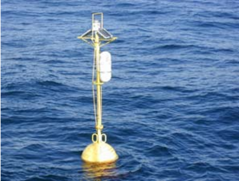
Figure 2. Showing spar buoy as deployed with light and radar reflector 10 ft. above the water level.
